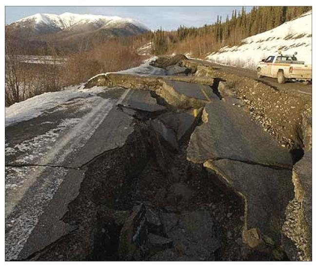
This rupture of the Tok Cutoff Highway in Alaska resulted from a magnitude 7.9 earthquake along the Denali Fault in 2002. The earthquake disrupted roadways and triggered thousands of landslides, but because of the sparsely populated terrain, no one died. (Courtesy Alaska Department of Transportation and Public Facilities)
